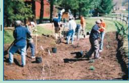
together. As you compress the soil, smooth it into a gradually rounded berm. This will be visually pleasing and also help reduce the erosion of the berm. Seed and straw the area with your choice of grass seeds. To prevent erosion prior to the establishment of grass, you may chose to place burlap or other matting on the berm.
